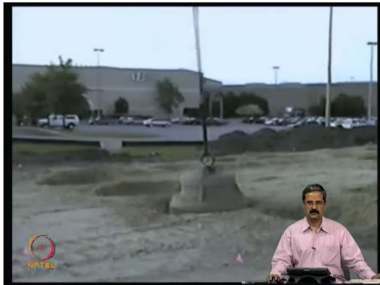
You can see that it is being done next to a shopping complex ((noise 00:37 to 02:41)). So, what you have seen is that it is a compaction using dynamic methods, where you try to compact as much as 10 meters of the in-situ soil and improve its performance.
