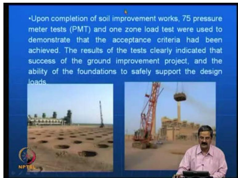
You can see that upon completion of the soil improvement this is a type of work that they have undertaken this from the particular company. They have done 75 pressuremeter tests and load test to demonstrate that the acceptant criteria had been achieved say for example, the acceptance criteria is what the bearing pressure and settlement.
