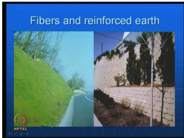
Another classic case is like fibers, fibers is another one that you can just use many of the fibers that is available like, people are used to fiber reinforced concrete, you can have fiber reinforced soil this is what actually the slope made of fiber reinforce soil. And fibers can be, they can be right from coir fibers, jute fibers then they can be even natural like the steel fibers, it depends on the application.
