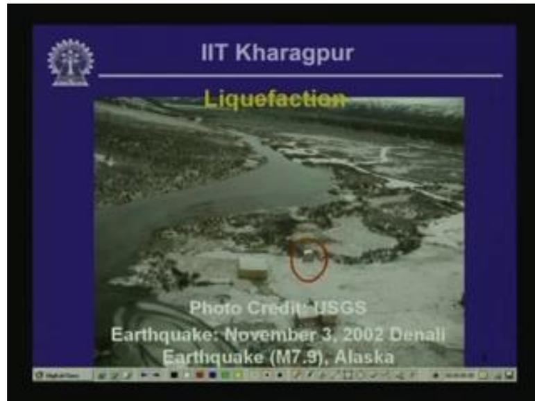
This structure was pushed up unevenly, and the cause of that is liquefaction and flotation that results from liquefaction, okay.
