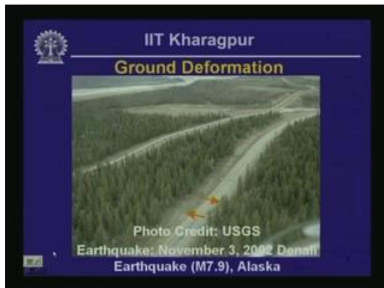
Now the fault movement took place like this. This was the sense of motion, and as I mentioned, the roller supports are in that area of the pipeline to account for this type of fault movement that largely mitigated the problem, but still there were some minor damages to the pipeline, okay.
