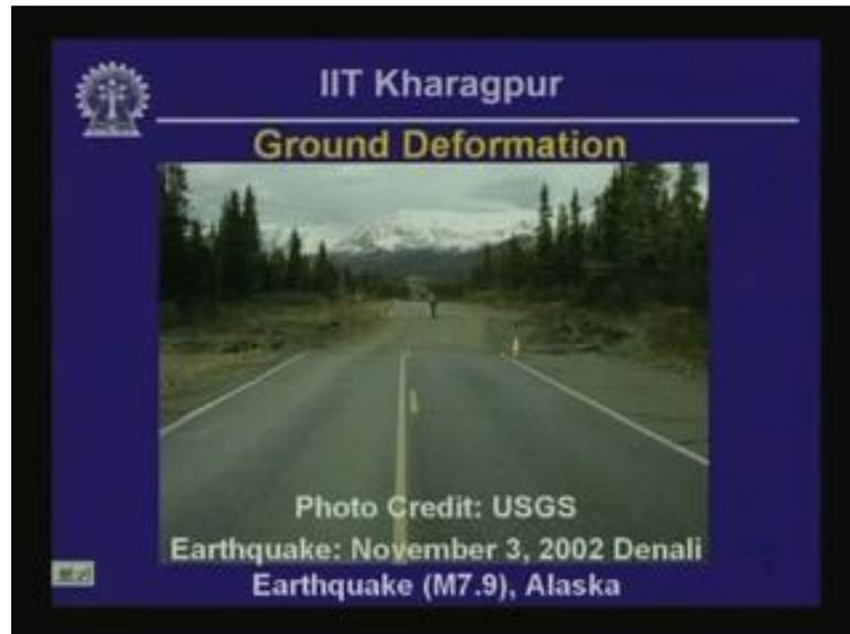
This shows a close up of the damage that we looked at in the aerial photograph shown in the previous slide. And here you can see the fault movement or the damage caused by the fault movement more clearly from the alignment of the central line marking or the divider marking of this particular highway.
